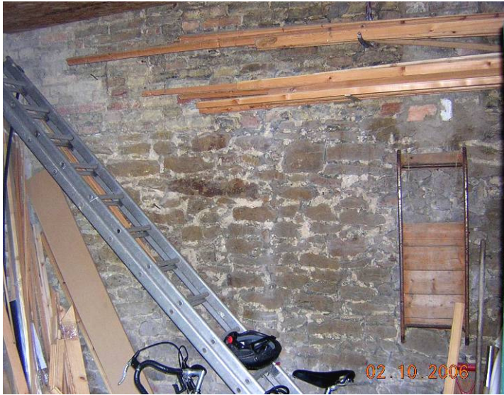
BACK WALL OF BRICK SHED
