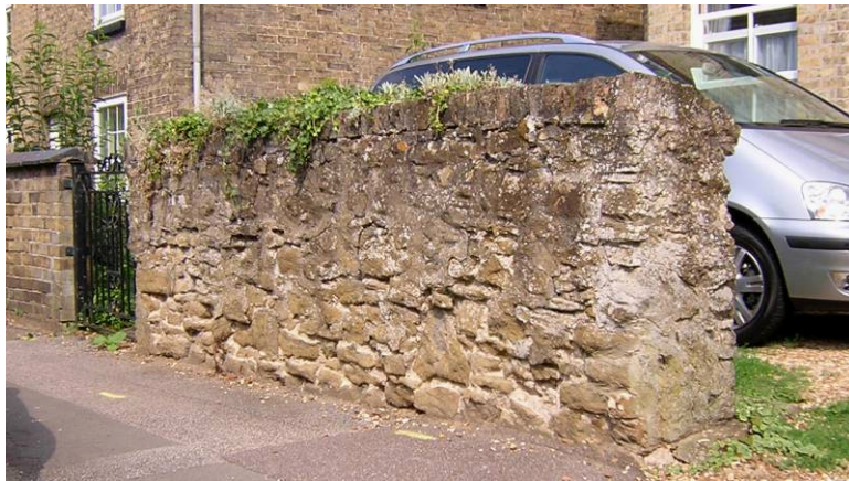
VIEW OF WALL 27
