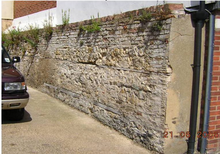
VIEW OF WALL 45
