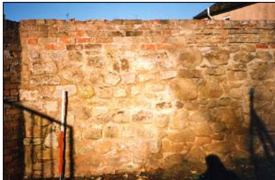
Figure : V 7R. Church Lane. Kings school. Viewed from east. Section 1
