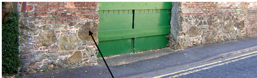
VIEW OF WALL 23
