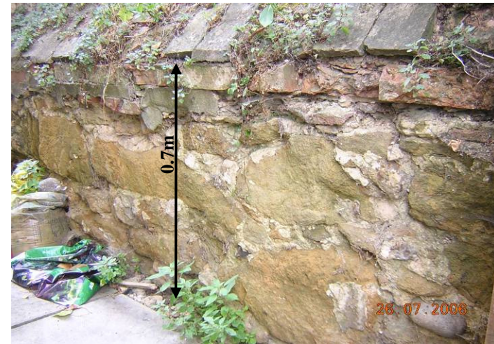
PART OF WALL 26
