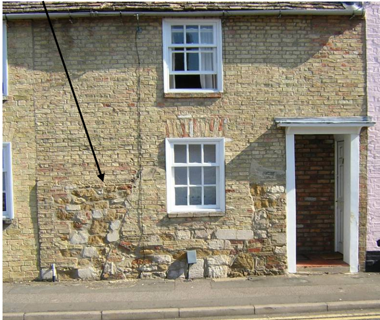
VIEW OF WALL 33
