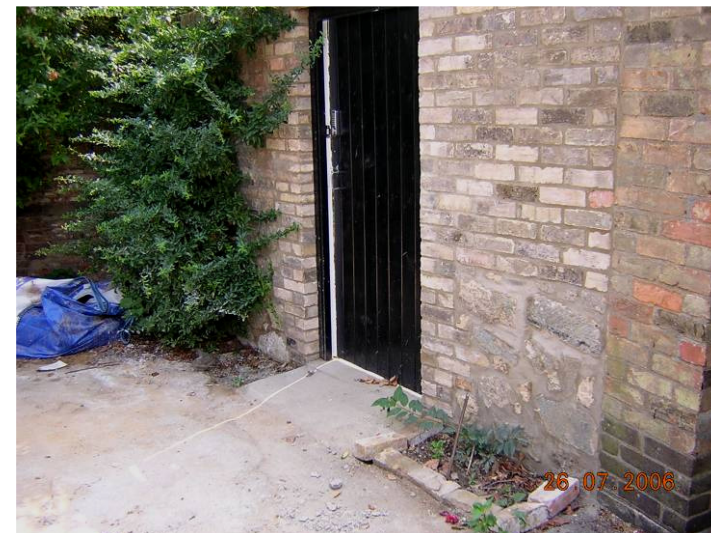
VIEW OF WALL 36
