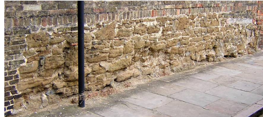
VIEW OF WALL 12
