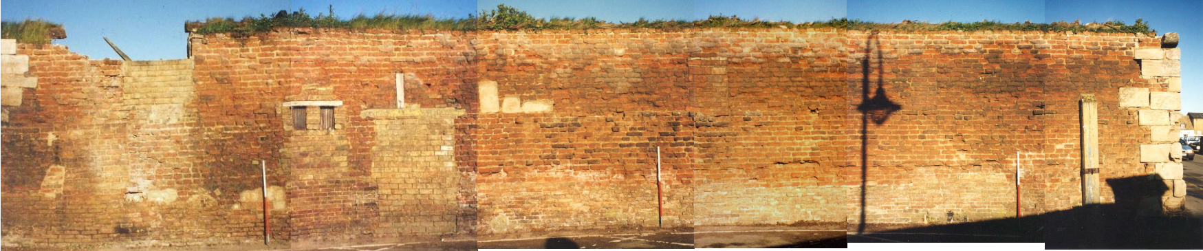
VIEW OF WALL S3A
