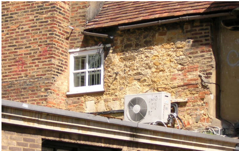
VIEW OF WALL 05
