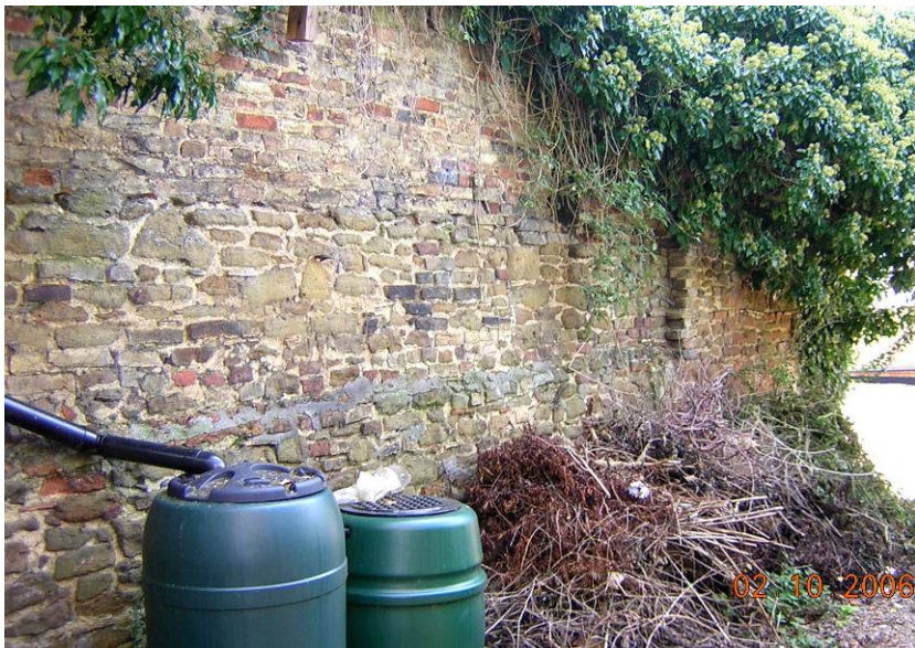
PART OF WALL 25
