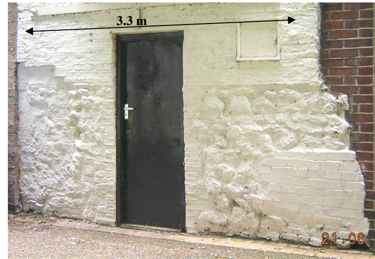
VIEW OF WALL 02
