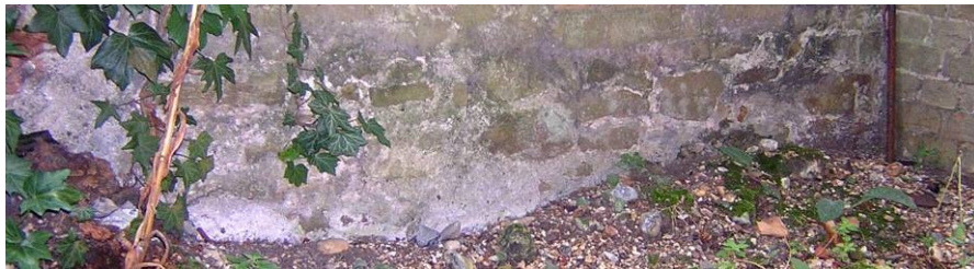
VIEW OF PART OF WALL 13
