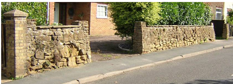
VIEW OF WALL 8
