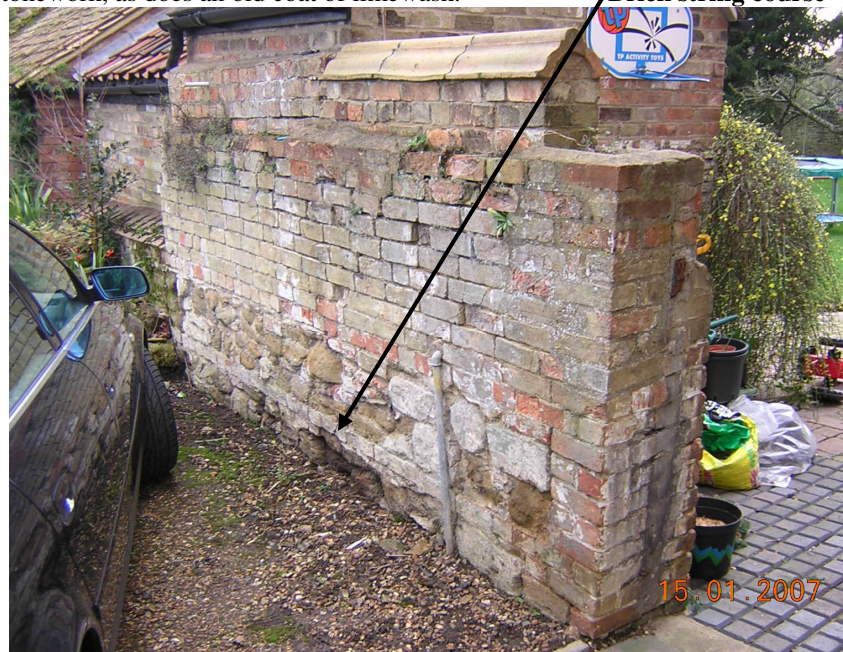
VIEW OF PART OF THE NORTH FACE OF WALL 30
