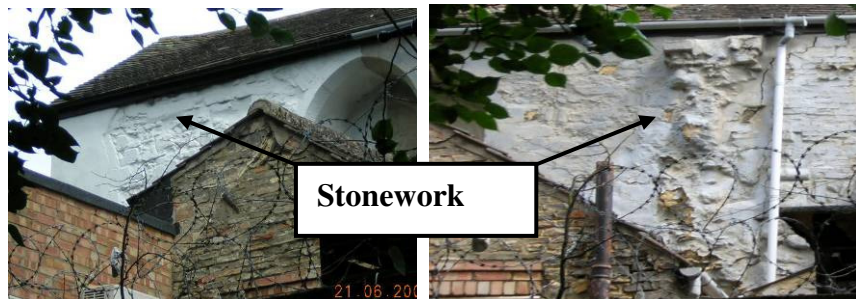
TWO VIEWS OF WALL 03
