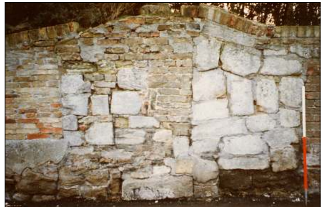
Figure : V 48. West End. Part of wall to St. John's Farmhouse
