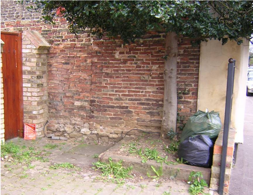
Wall showing stonework at base and pre 1725 brickwork above.
