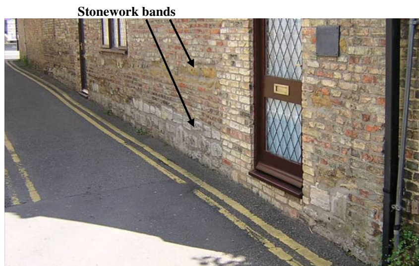
VIEW OF WALL No 07
