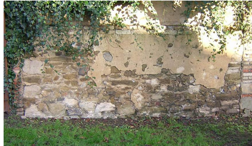
VIEW OF WALL 8
