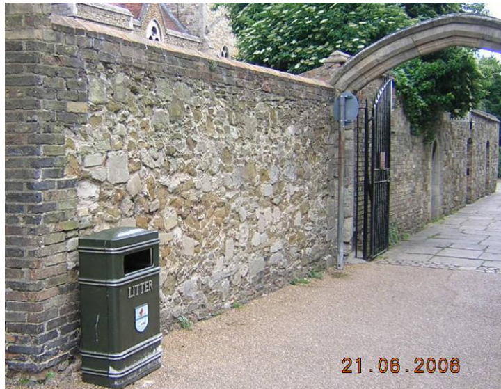
VIEW OF WALL 01
