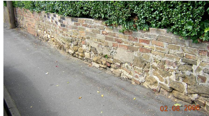
VIEW OF WALL 56
