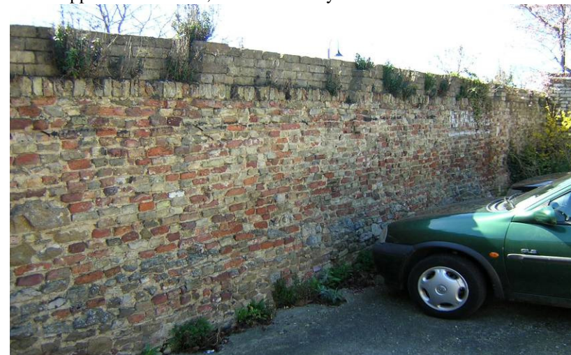
VIEW OF PART OF WALL 54
