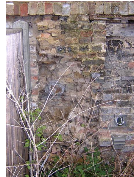
VIEW OF WALL 6
