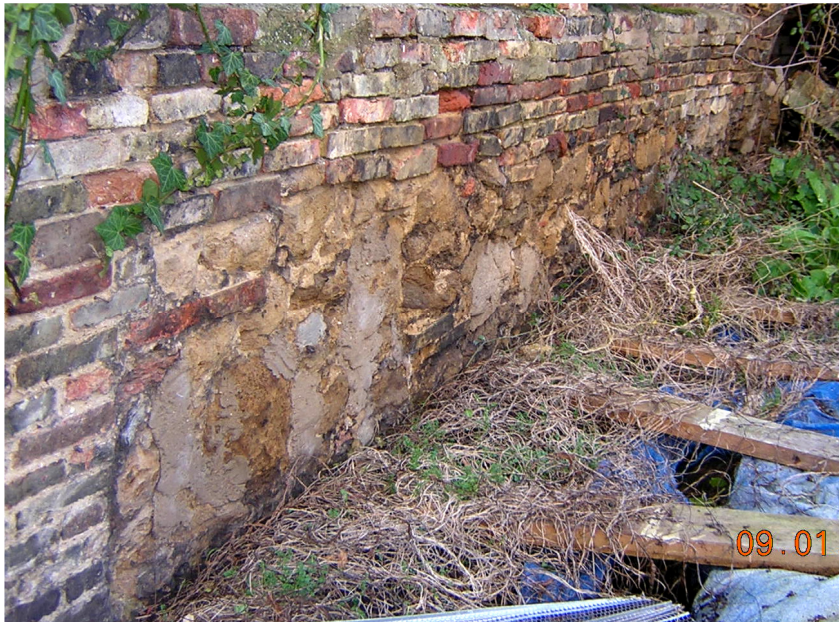
PART OF WALL 15
