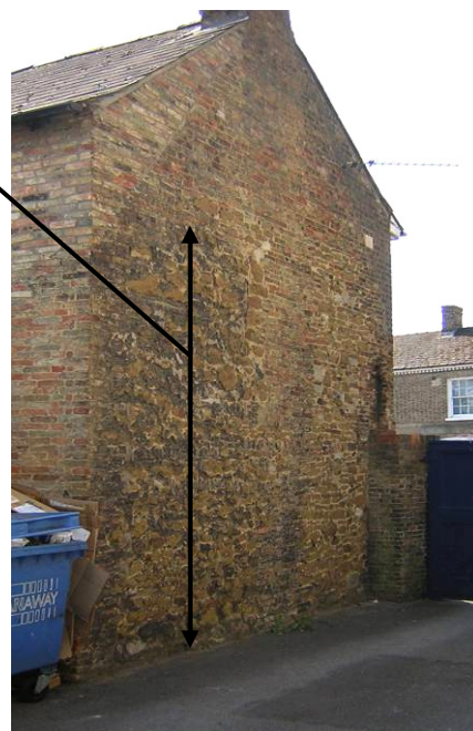
VIEW OF WALL 17
