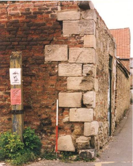
CORNER OF WALLS S3A and S3B
