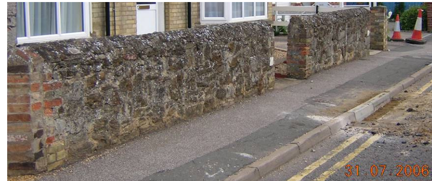
VIEW OF WALL 40
