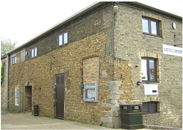
VIEW OF WALL No 21
