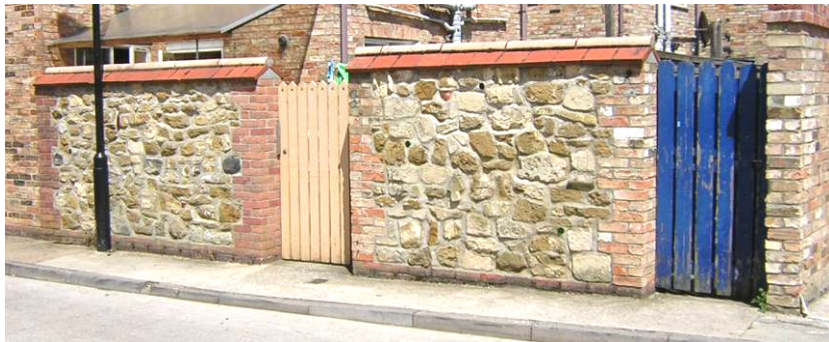
Above: VIEW OF WALL 51
