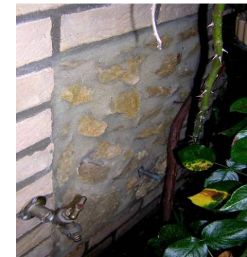
NEW STONE PANEL
