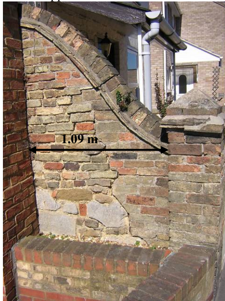
VIEW OF WALL 57
