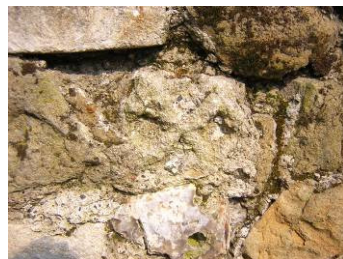
Right: A DETAIL OF WALL 53
