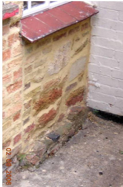
VIEW OF WALL 31
