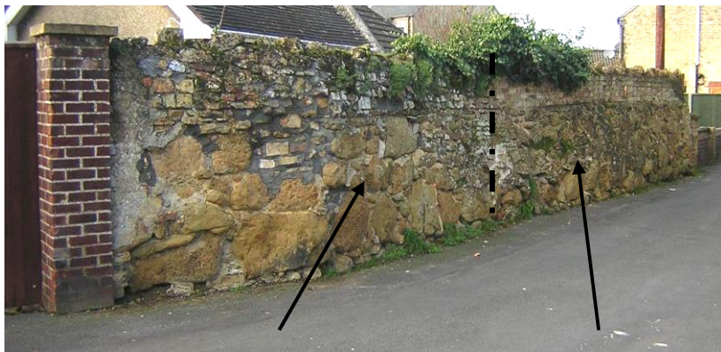
Wall 17 C Wall 17 D VIEW OF WALL 17 C AND 17 D
