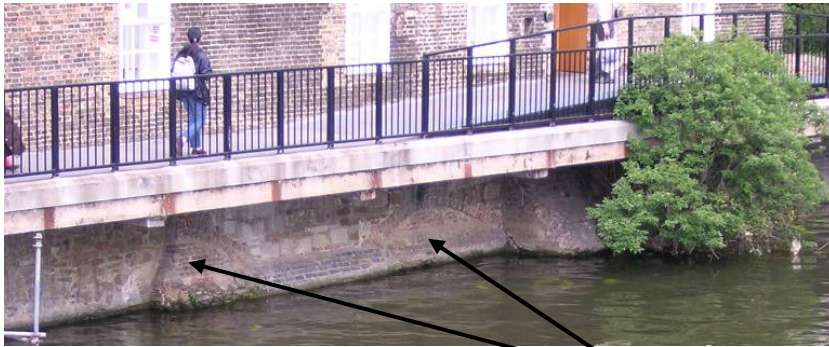
VIEW OF WALL No 25
