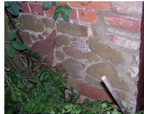
PART OF WALL 30
