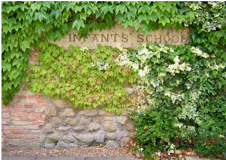
VIEW OF PART OF WALL 43
