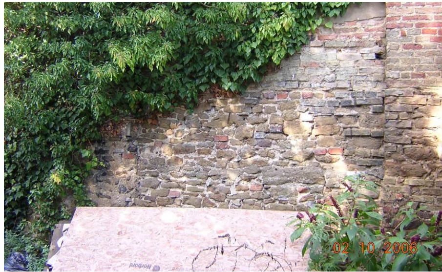
PART OF WALL 24
