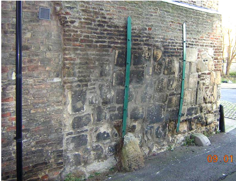
VIEW OF WALL 9
