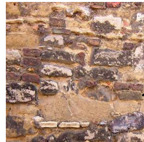
DETAIL OF STONWORK
