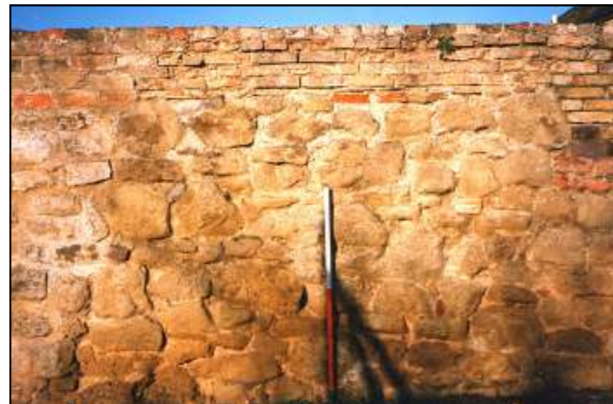
Figure : V 7R. Church Lane. Kings school. Viewed from east. Section 2
