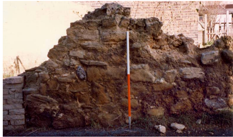
VIEW OF WALL 19
