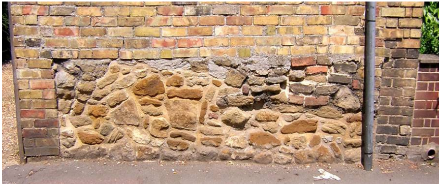
VIEW OF WALL 25
