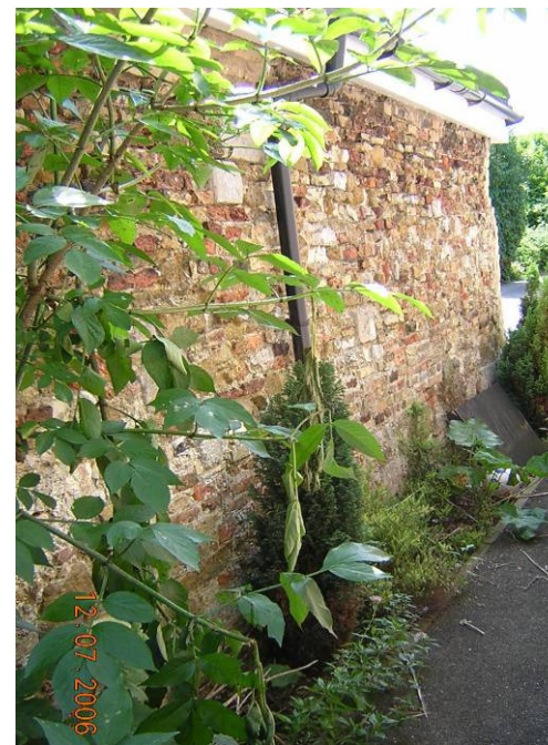
VIEW OF PART OF WALL 20
