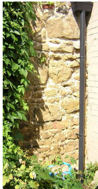
VIEW OF PART OF WALL 29
