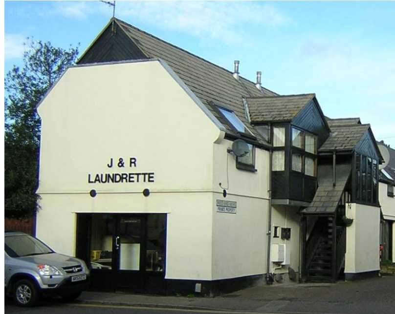
General view of building after the render was applied.
