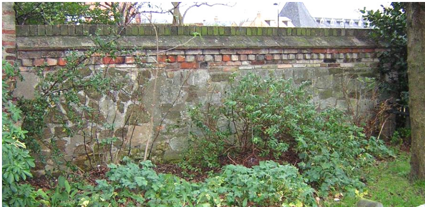
VIEW OF WALL 11 FROM JUBILEE TERRACE
