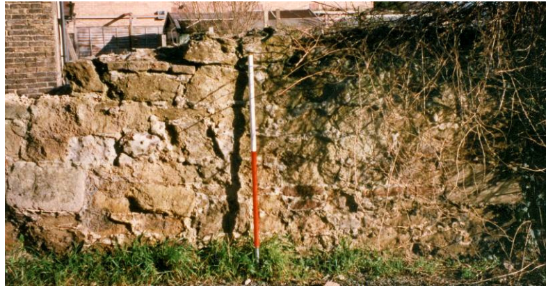
VIEW OF WALL 18
