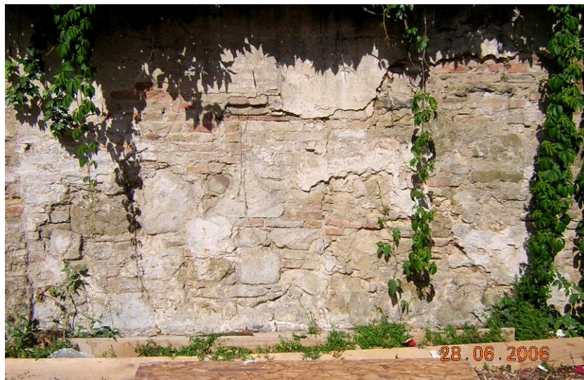
VIEW OF INNER FACE OF PORTION A
