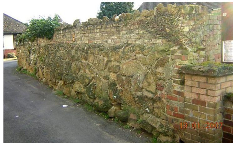
VIEW OF WALL 17D
