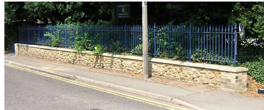
VIEW OF WALL 38
