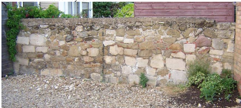
Above: VIEW OF PART OF WALL 53
