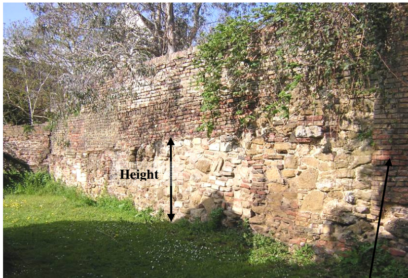
VIEW OF WALL No 13
