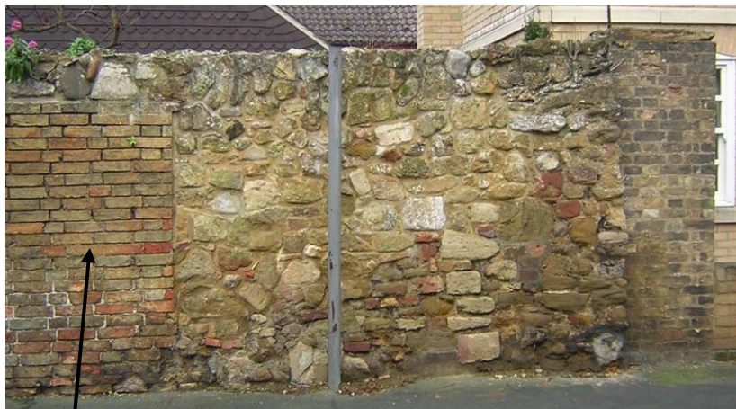
VIEW OF WALL 12A
