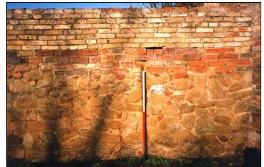
Figure : V 7R. Church Lane. Kings school. Viewed from east. Section 3
