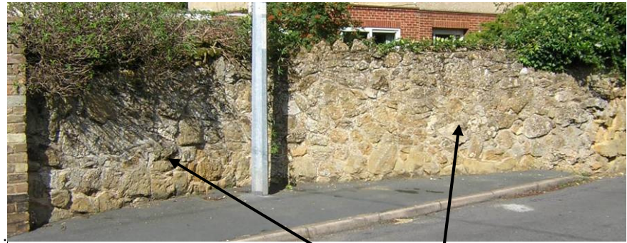
VIEW OF WALLS 16B AND 16C
