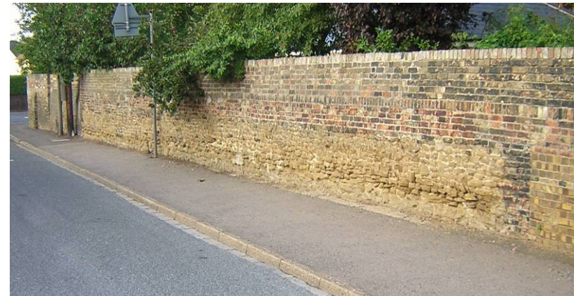
VIEW OF WALL 34
