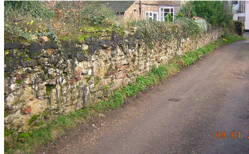
VIEW OF PART OF WALL 16
