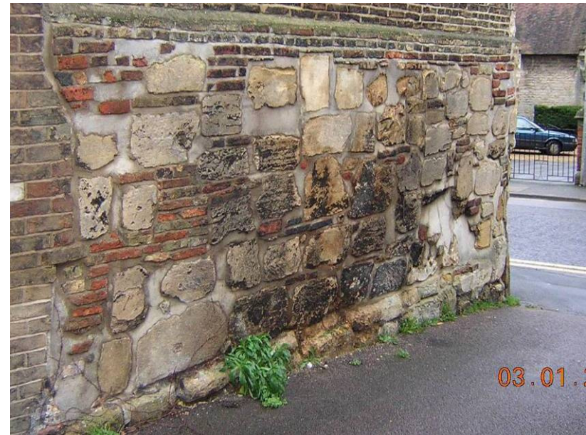
VIEW OF WALL 12
